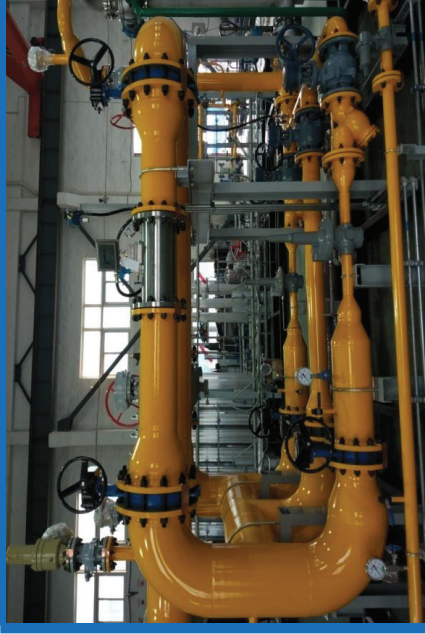
N2 Gas Measurement On Site
